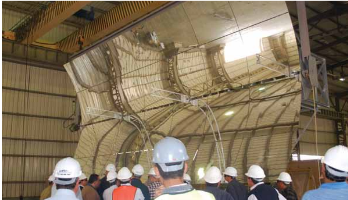
Parabolic trough reflectors for the WBG/GEF-financed Al-Kureimat solar thermal power plant in Egypt being assembled, March 2009.
