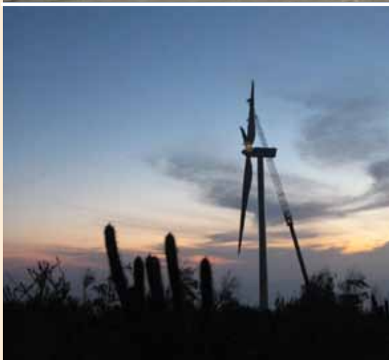
Construction under IFC-funded SN Power/Centinela wind project in Chile.
