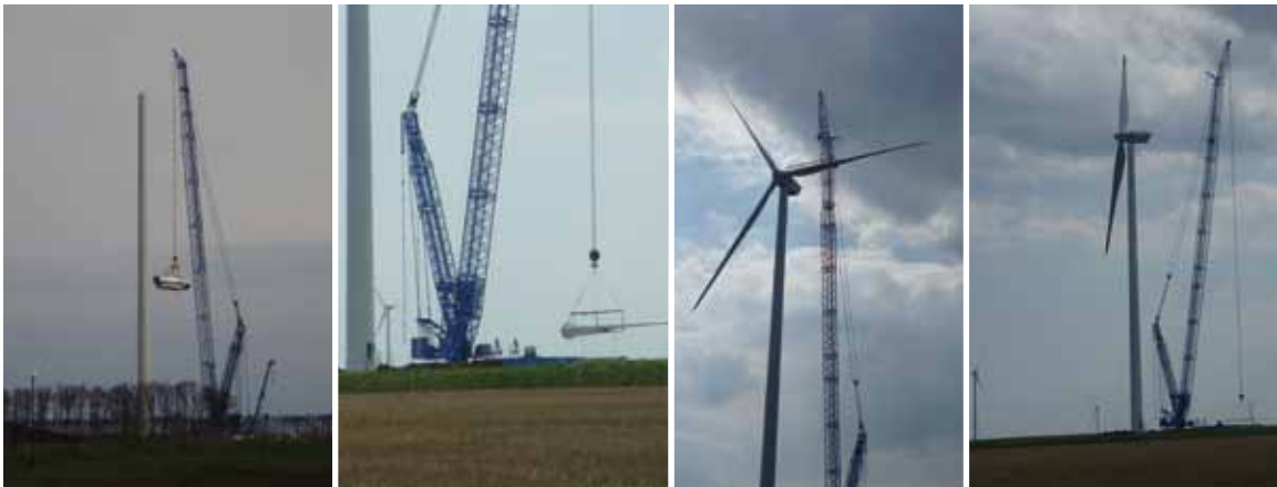
Construction of the 156 MW St. Nikola Wind Farm in the municipality of Kavarna, in the north-east of Bulgaria, on an elevated plain approximately 3km from the Black Sea (IFC project, "AES Kavarna"). The wind park comprises 52 3 MW V90 turbines, manufactured by Vestas A.S. (Vestas) of Denmark. The project includes a 33/110 kV substation, connected to the national grid through an 8 km transmission line.
