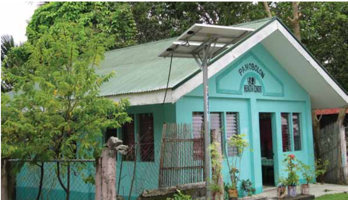
Panabolon Health Center, Philippines; electrified under the World Bank/GEF-assisted Rural Power Project.
