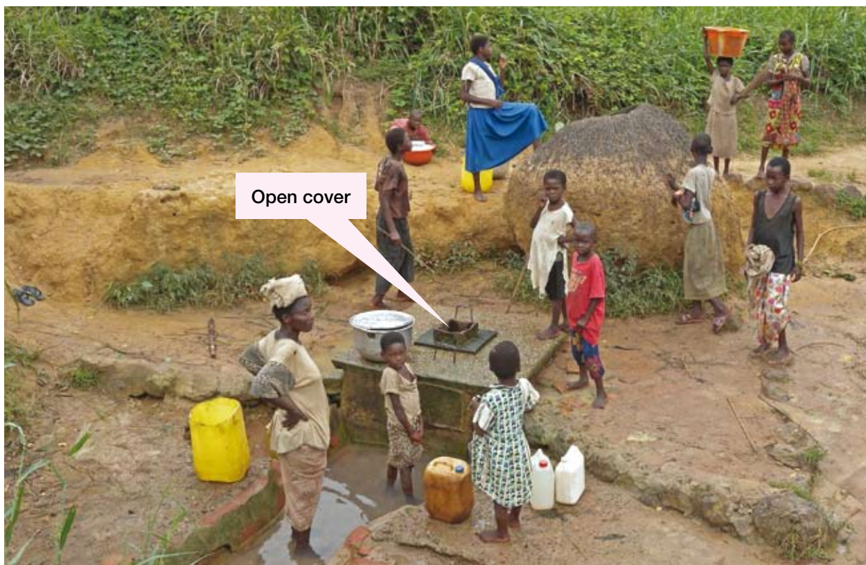
The protective cover of this spring box is partially exposed rendering contamination inevitable. Note also the lack of any diversion ditch and fence around the site to protect from pollution. (Denge spring, Libenge, Equateur Province)
