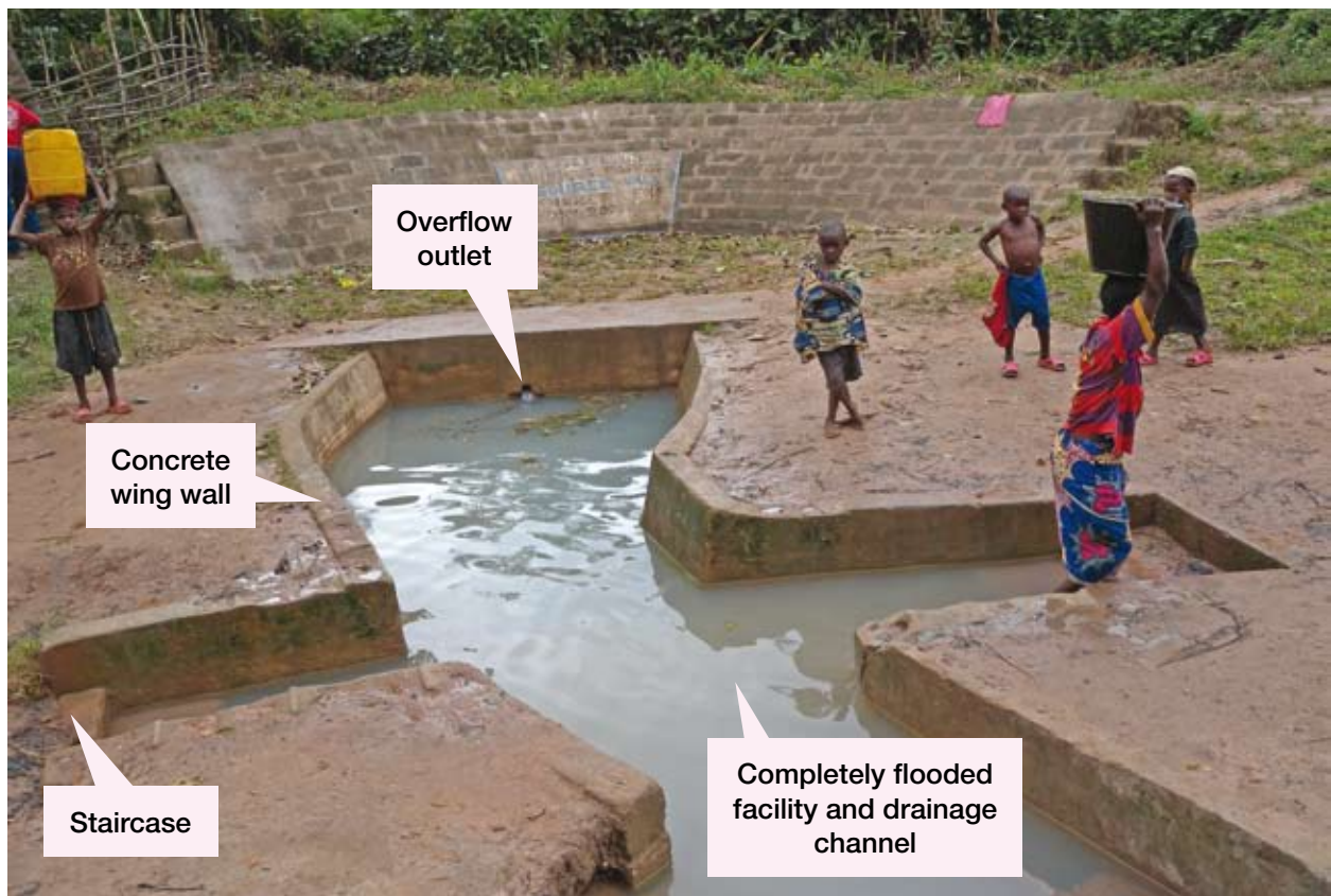
Constructed in July 2006, the Vala spring box in Libenge, Equateur Province, fell into disrepair by 2008, forcing local communities to tap seepage around the spring box or travel longer distances in search for water
