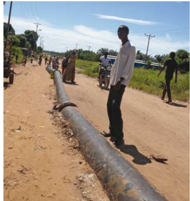
REGIDESO's main transmission pipeline in Mbuji-Mayi is exposed to a high risk of structural deterioration. This occurred in February 2010 when a catastrophic failure caused the sudden loss of millions of liters of water and damage to surrounding property. Water delivery was cut-off for several weeks in this city of over one million residents (above and below)
