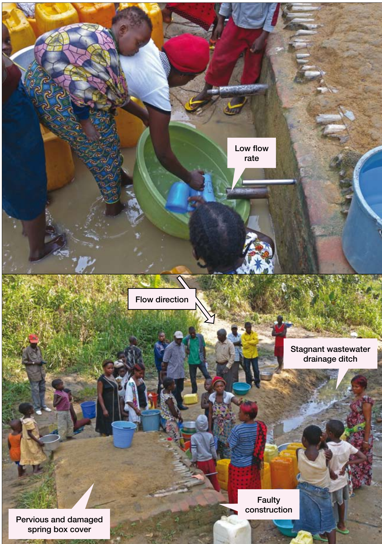
In Kalima, Mainema Province, the Baganda spring box combines several features of poor construction and maintenance including: reduced flow rate, damaged spring box cover, sediment build-up and clogging of the drainage ditch, lack of fence enclosure and upslope footpaths increasing erosion and contamination risks
