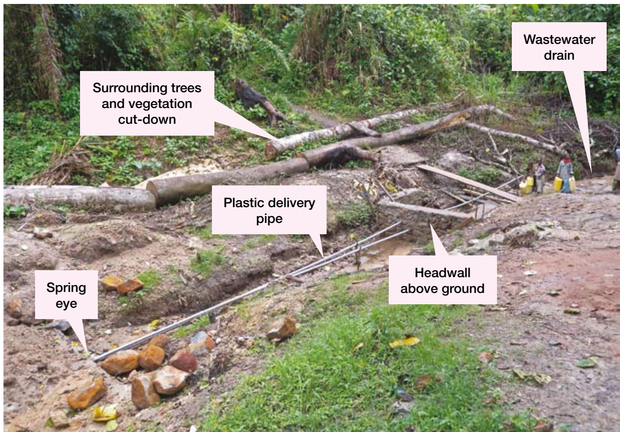
Work in progress: construction of a retaining headwall in the village of Kandate in Ituri District
