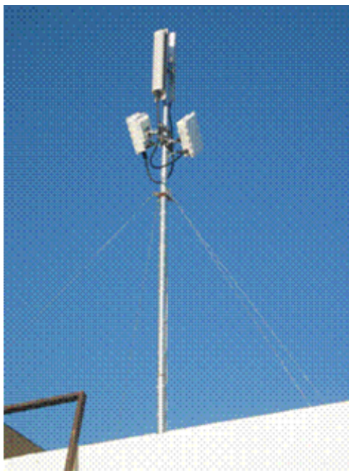
Figure Anx 3.25: Typical WiMAX installation, with two base stations linked to two 60 degree sectored WiMAX antennas
