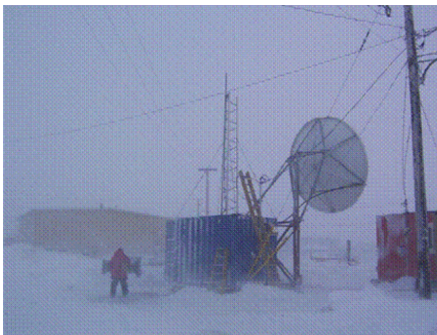
Figure Anx 3.18: QINIQ Network: Installation of 4.5 m antenna, communications shelter and wireless tower at Gjoa Haven, Nunavut, at 68° North
