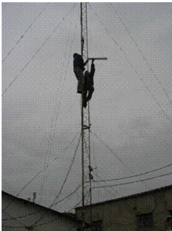
Figure Anx 3.4: Installation of Yagi (directional) antenna
