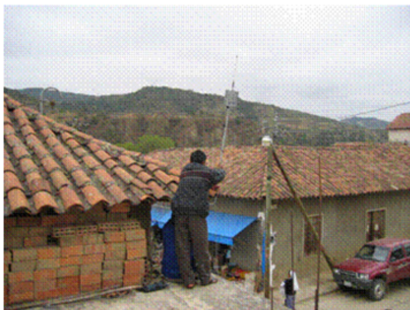
Figure Anx 3.5: Installation of a mesh box at the telecenter, Sopachuy (The omni-directional antenna is located on top of the mesh box)
