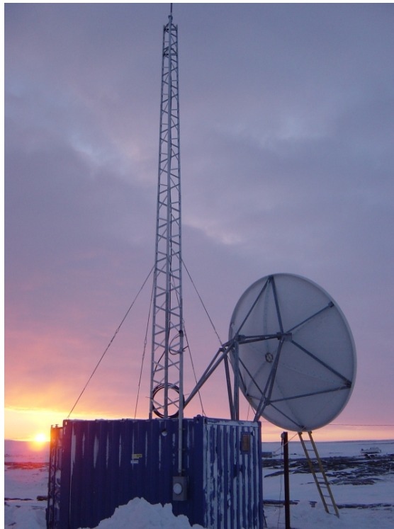
Figure VII.4: QINIQ Network: 4.5 m. VSAT, Base Station Antenna Tower and shelter at Chesterfield, Nunavut, Canada
