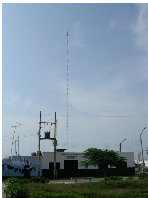
Figure VII.5: Tower and Yagi Directional Antenna of the Chancay-Huaral WiFi backbone network, at the farmers' cooperative in La Huaca, Peru
