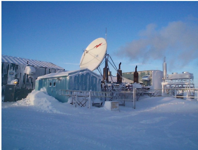
Figure VII.3: QINIQ Network: 4.5 m. VSAT Antenna at Arviat, Nunavut, Canada
